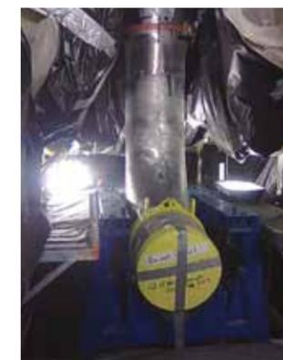
Three years ago, as part of the new construction of a third reactor in Olkiluoto, Finland, INSPECTOR SYSTEMS was awarded the contract to grind the various primary circulation pipeline system welds which were of relevance to safety from the inside. For this a number of grinding robots and exhaust robots were developed, built and qualified for the relevant diameters ranging from DN 100 to DN 500.
